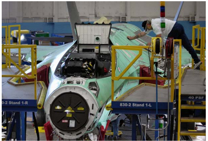
Lockheed and its suppliers are identifying the causes of reliability problems with F-35 components, said J.D. McFarlan, vice president of F-35 testing. New parts are designed and produced and are installed as soon as they are available, and planes are returned to testing.
